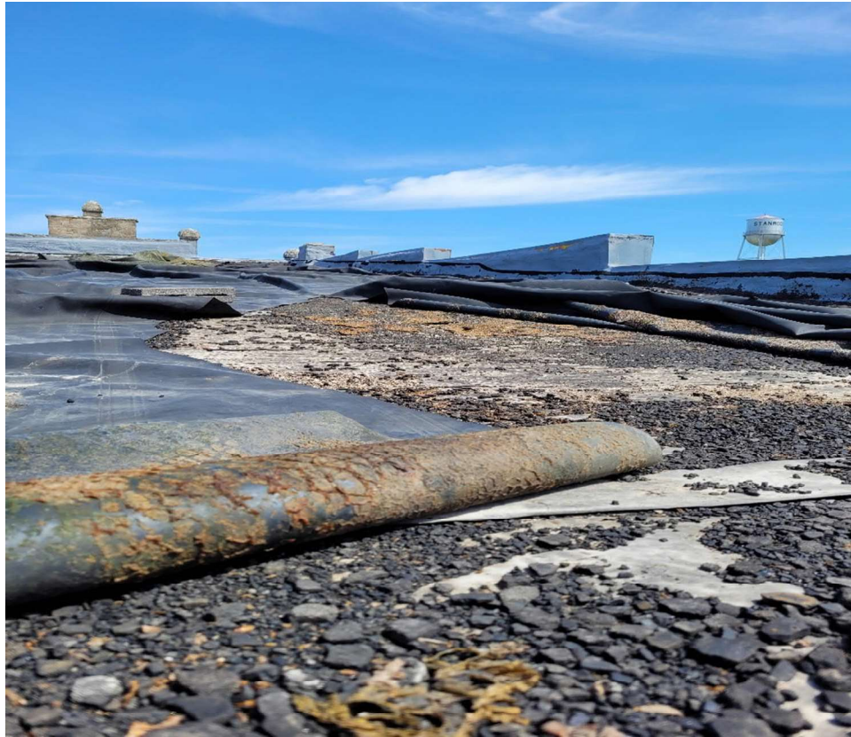
Photo 9: View of positive roof decking and flashing throughout both building roofs.
